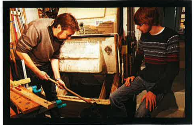
Test case one: in Hamburg's ecological settlement of Allermöhe, solid, liquid and paper from the dry toilet drop into a compost tank in the basement.
